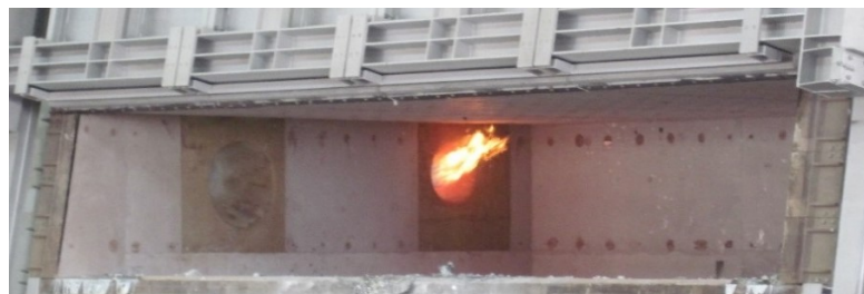
Figure 2. Reverberatory gas-fired metal holding furnace
