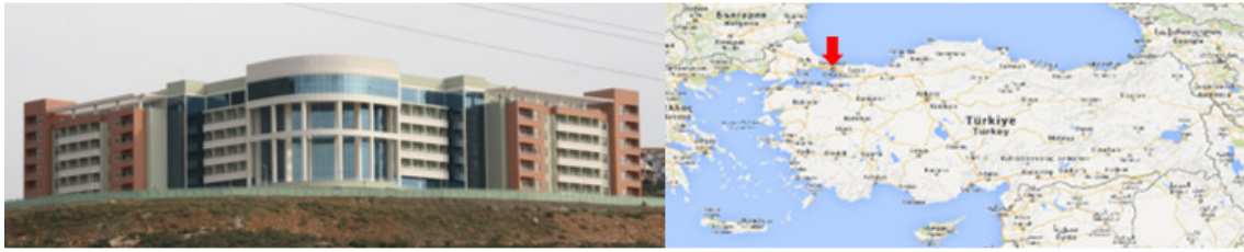
Figure 2. The front view of the building and the location of the building
