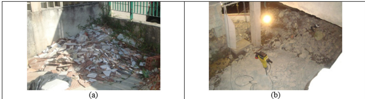
Figure 2. Construction waste (a) and demolition waste (b)
