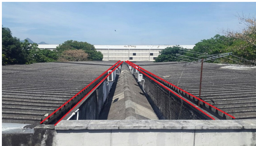
Figure 7. Rainwater gathering – existing gutters
